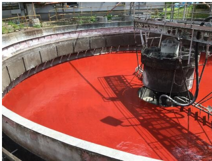
MasterSeal 7000 CR in sedimentation tank in WWTP Harmanec, Slovakia
